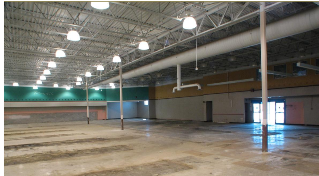
East Interior Space Shown – Front Half
